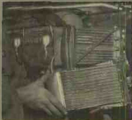
The old oil cooler, shown below the new installation.
